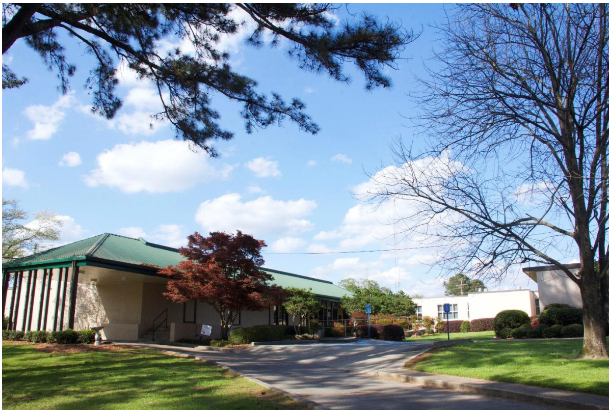
PHOTO: Jefferson Davis Community Hospital, Courtesy of Forrest General Hospital
